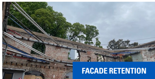
CRANE BACK PROPPING
